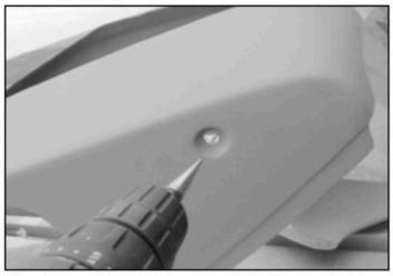
Using a uni bit, drill the center of the upper and lower mounting bosses to the desired width hole. Measure twice, drill once!
